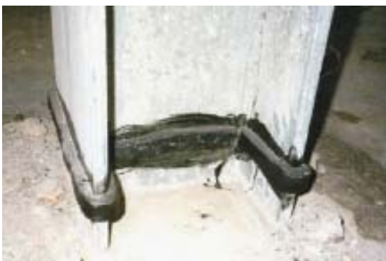
Installed Contite Waterstop Around King Post
