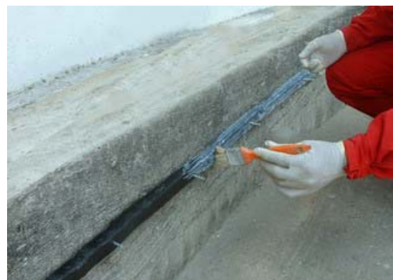
Contite Waterstop Delay Coating application by brush
