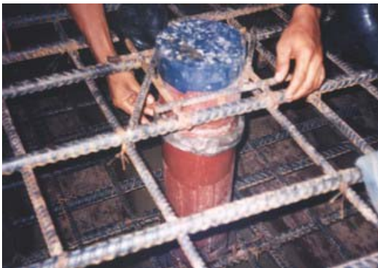
Installing Contite Waterstop Around Pipes
