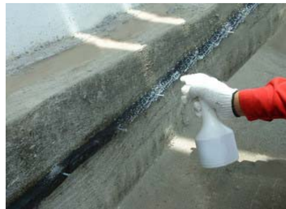
Contite Waterstop Delay Coating application by spray
